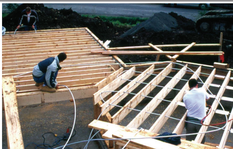
Ultra-Fin Radiant Floor Heating System installed from above
